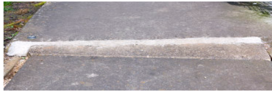
tripping hazard - repaired
